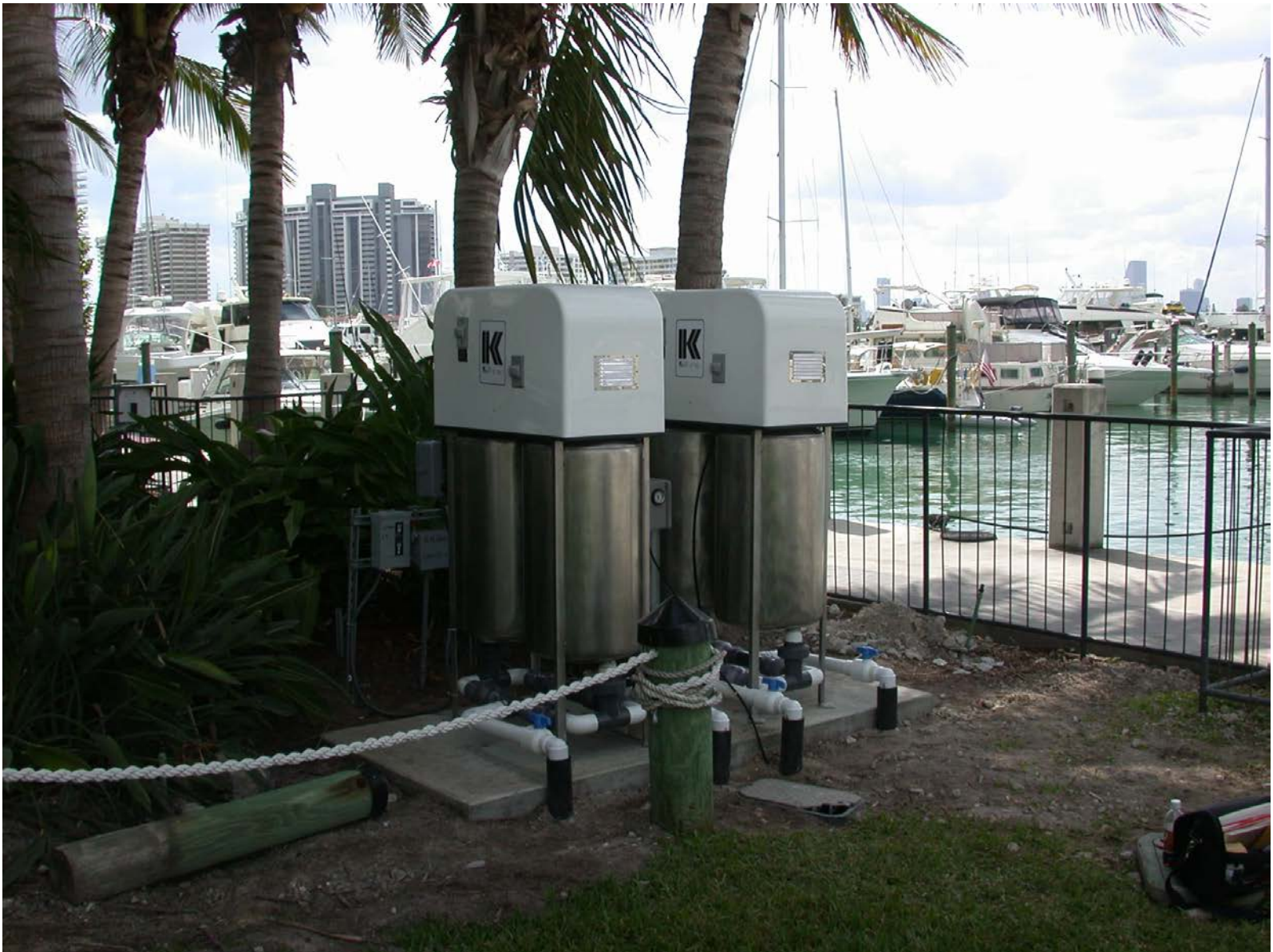
Vacuum Type System, Sample Landside Installation
