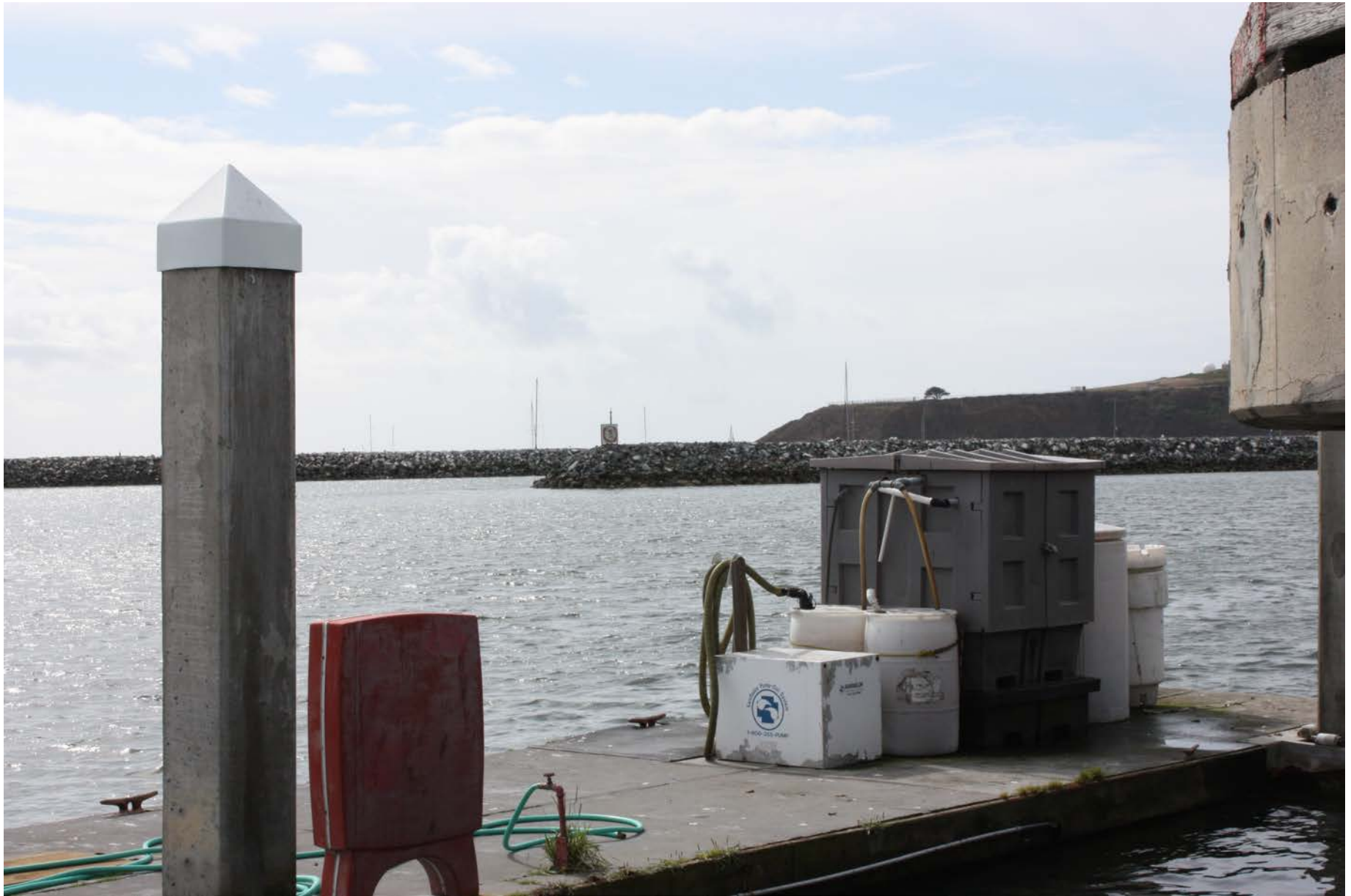
Don't : DIY – Oil Water Separator
