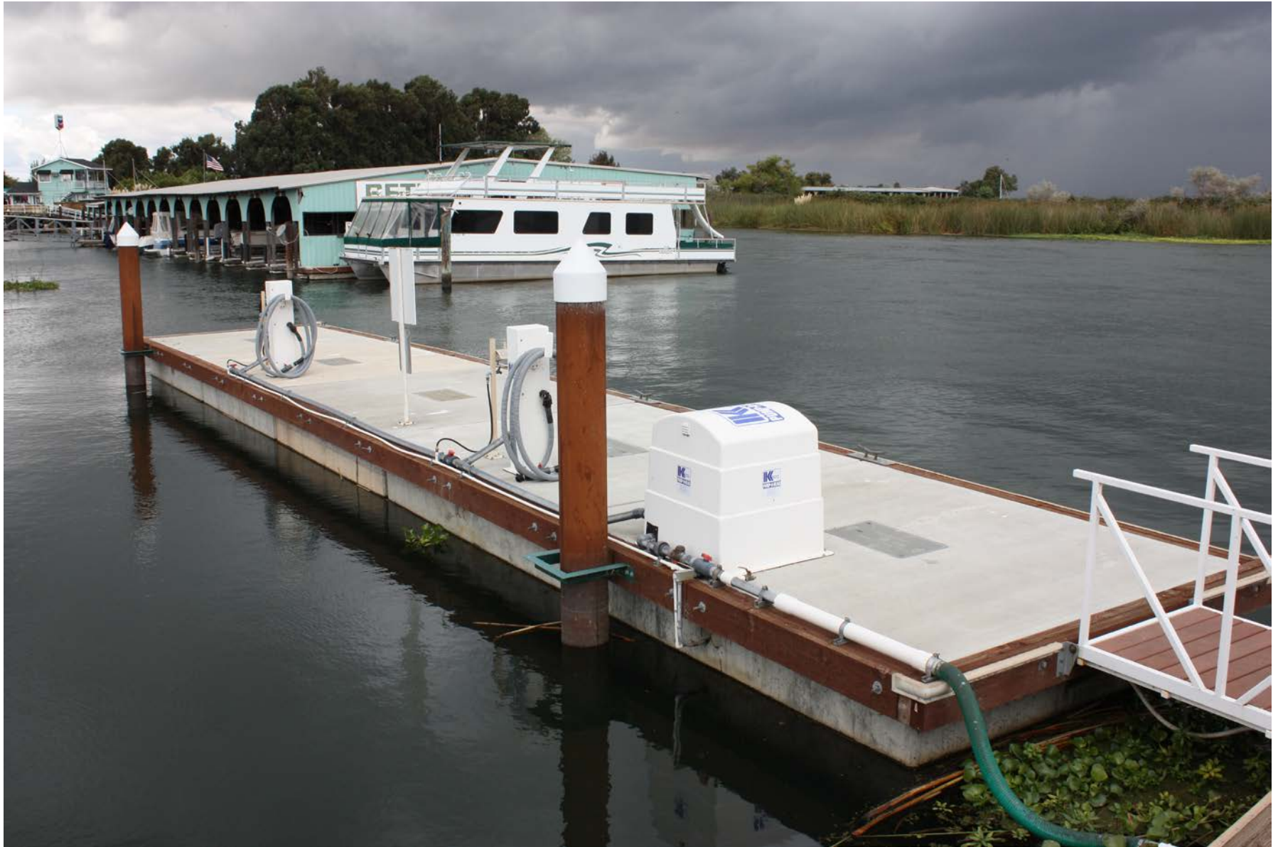
Do: Dedicated PumpOut Dock
