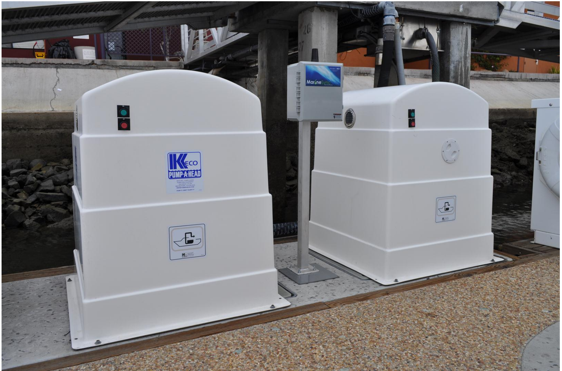
Peristaltic Type System, Sample Dockside Installation
